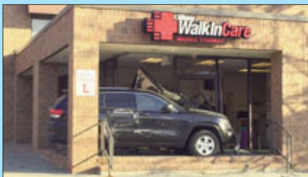
Gunderland, NY: A car crashed into Albany Walk-in Care after the driver accidentally hit the gas instead of the brake. Nobody was injured. Photo courtesy of News10 ABC, Albany, NY ( http://news10.com/2017/01/16/car-slams-into-albany-urgent-care-building/ ).
